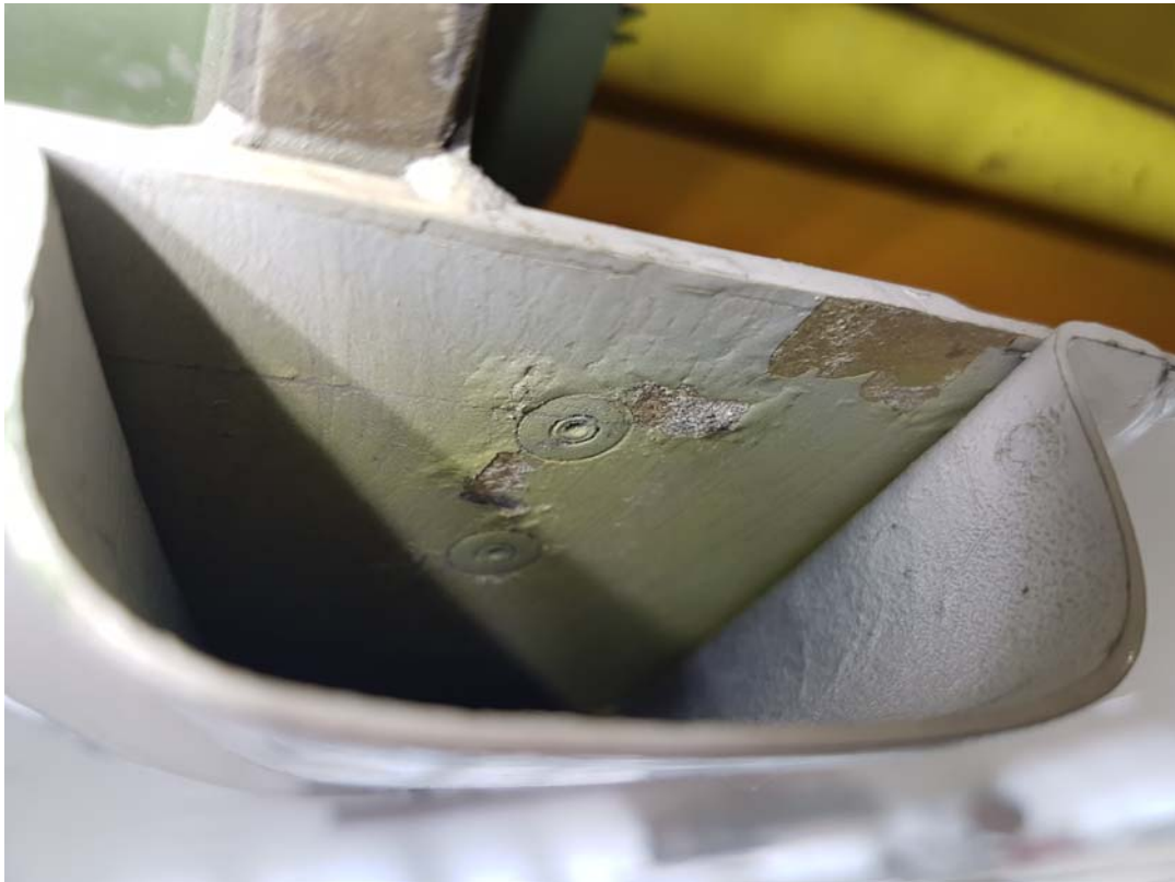
Figure 6. Example of Damage - Mid Forward Flap Track Fairing
