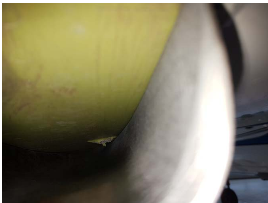
Figure 5. Example of Damage - Outboard Forward Flap Track Fairing
